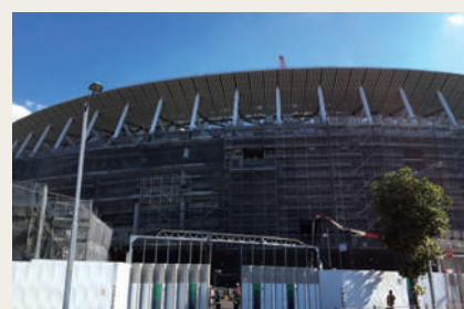
The Olympic Stadium under construction
